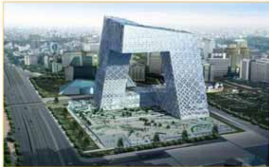
中央电视台新台址 中央电视台新台址工程位于北京市朝阳区中央商务区（CBD）核心地带。中央电视台新台址用地面积总计187,000平方米，总建筑面积约55万平方米，最高建筑约230米。中央电视台新台址建设工程确定采用荷兰OMA的设计方案。专家评审认为这一方案不仅体现立CCTV的标志性形象，也将翻开中国建筑界新的一页。中国中央电视台新台址工程是建国以来国家建设的单体最大的公共文化设施。也是2008年北京奥运会的重要配套设施之一，并将成为北京市重要的标志性建筑。重要的文化景观。 联和强成功应用于中央电视台新台址中玻璃幕墙的伸缩与密封胶条，是联和强实力的展示。 The new CCTV building The new CCTV building was located in the core zone of central business district (CBD), Chaoyang District, Beijing. With a plot area of 187,000 sq. m and total construction area of about 550,000 square metres, the top of the building is about 230 meters. The new CCTV building project adopts the OMA design plan of the Netherlands. The expert judges think that this program will set up the CCTV image and open a new era for the Chinese construction field. The new Chinese CCTV building is the largest monomer public cultural facilities since the founding of China and one of important supporting facilities for the 2008 Beijing Olympics, and it will become an important landmark building and cultural landscape. The expansion and sealing rubber strip of glass curtain walls made by Lianheqiang for the new CCTV building displayed its strength.
